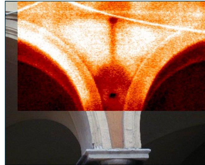
Investigation on hidden steel tie rods
