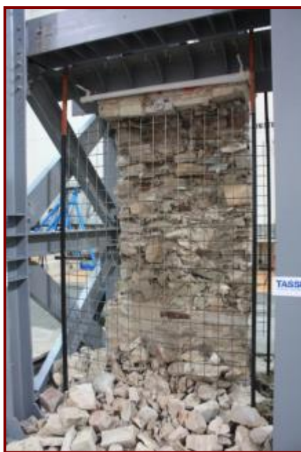
Unstrengthened condition 0.25g
